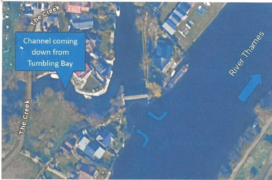
Figure 3 – Little Grey Weir (Source: Google Maps)
