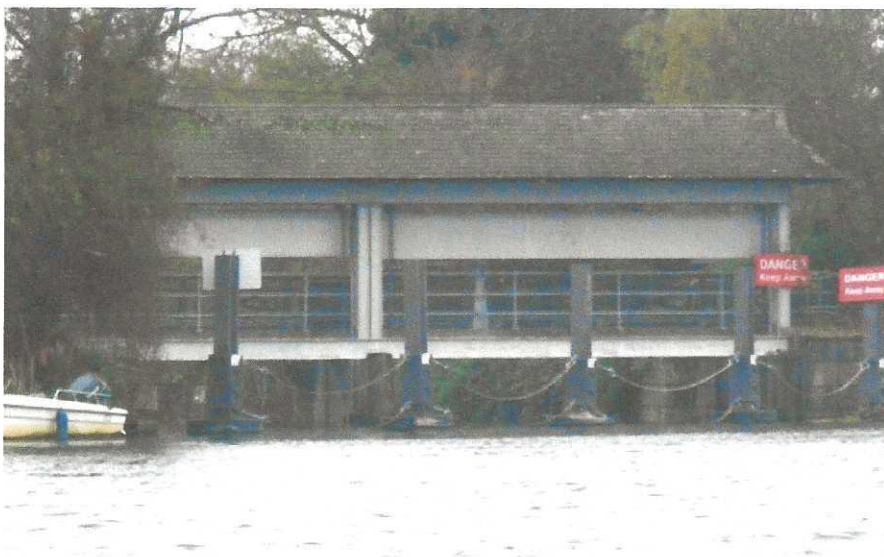
Figure 4 – gates closed (photo Mike Hendry)
